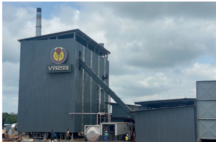
Project in Ghana: a full scope cogeneration plant for the growing energy demands of the palm oil mills and refineries of this palm oil producer
