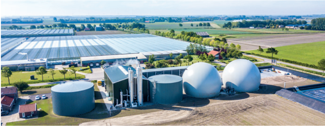
Project in The Netherlands: the first in the world to capture CO 2 derived from biomass on site and to inject it directly into the greenhouses as a locally sourced fertiliser
