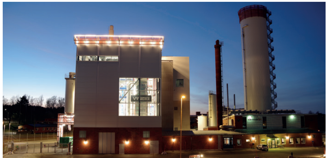
Project in Sweden: RDF-fired heat plant for Nordic energy provider. A turnkey superheated water boiler will process RDF and provide district heating to a network of approx. 2,500 homes in Säfte, Sweden
